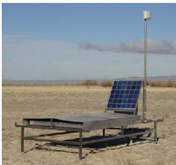
Fig. 11: A picture of a deployed SD. Scintillator box is under the roof visible in the picture. Electronics box is located under the solar panel. These components are on the iron frame.
