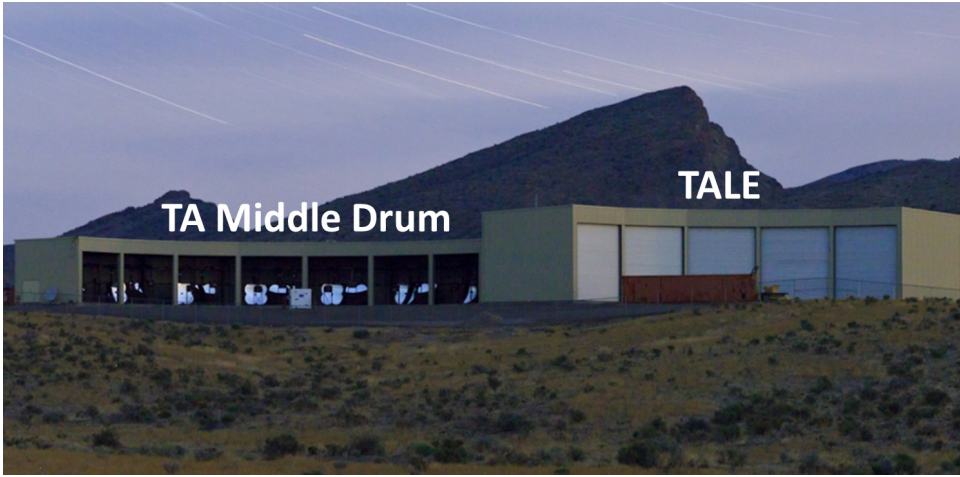
FIGURE 2.7: Photo of the TA MD (left) and TALE FD (right) building.
